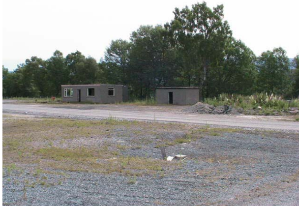
Fig. 4 : Existing derelict structures to the south of existing access road
